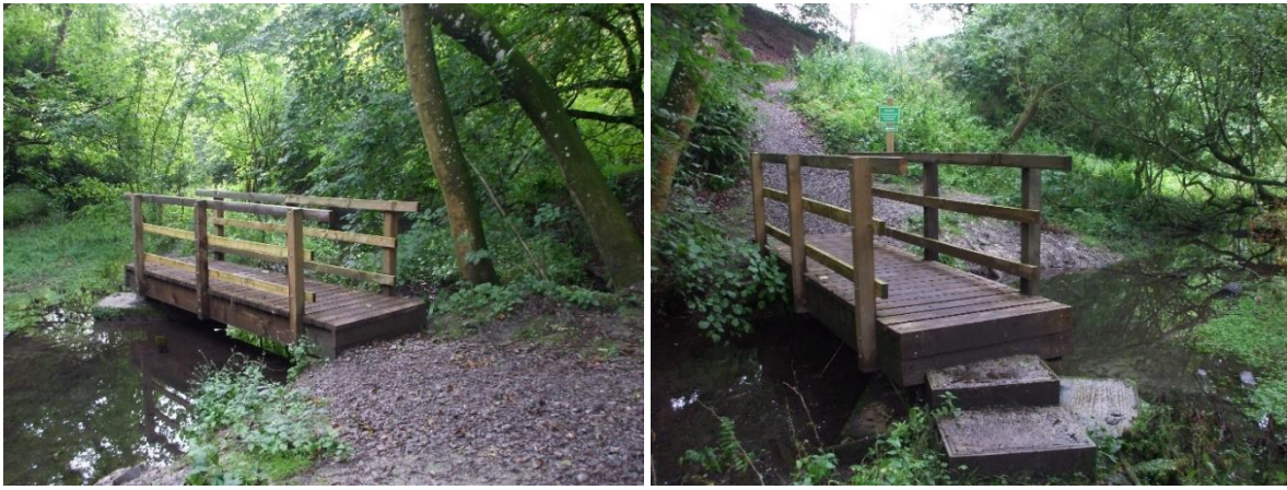
Sept 2020 the bridge is situated and the continuation point of the diversion
