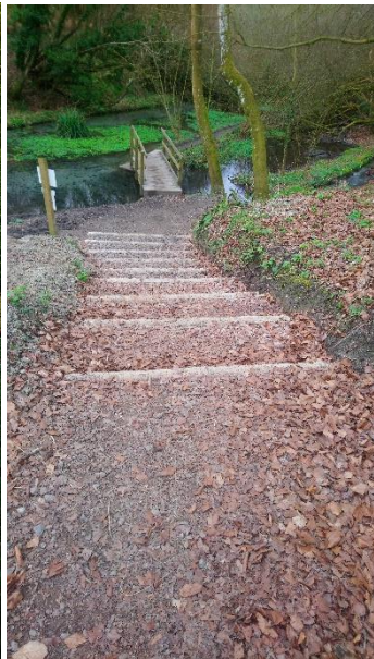
2021 following installation of steps
