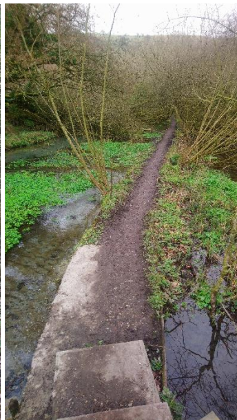
Mar 2021 showing clearance work
